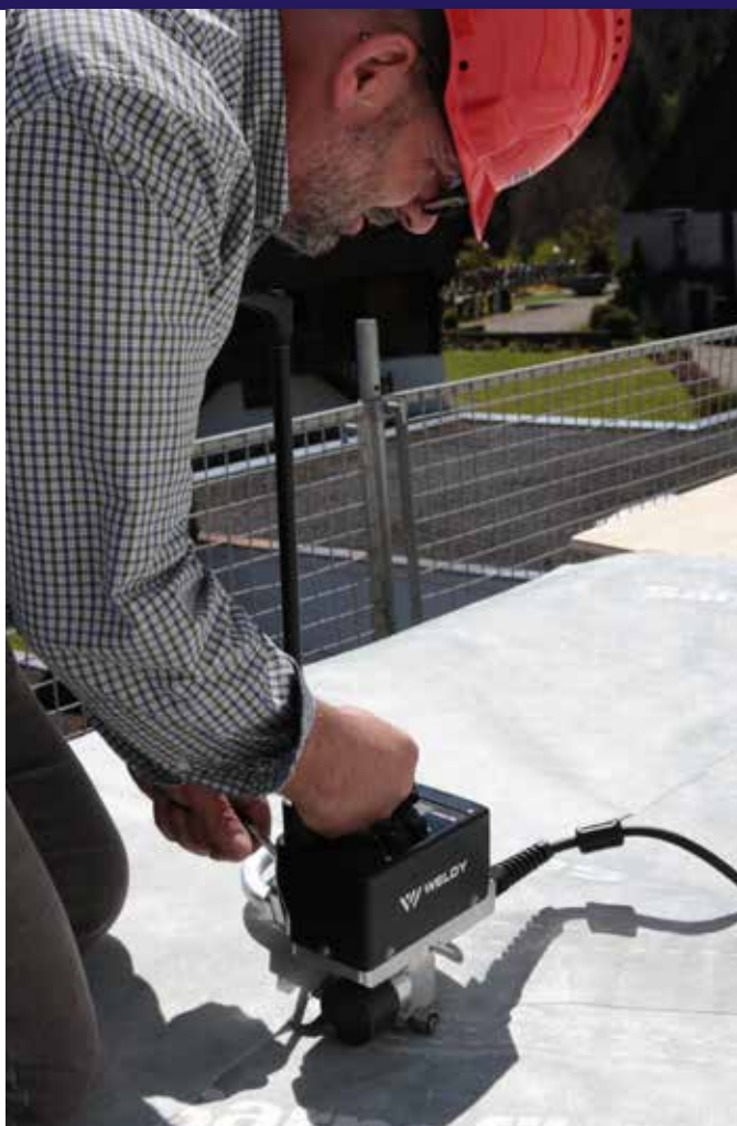
158.977 (230 V) 151.958 (120 V) Hot wedge, 40 mm Chromium steel (for PVC)
