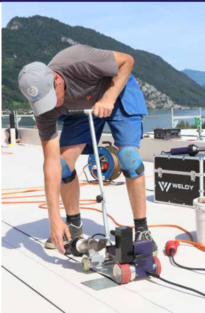
123.287 Overlap welding nozzle, 40 mm
